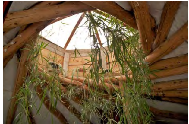
Below, typical Lammas round house, top left shows greenhouse extension and top right apex detail of reciprocal frame roof.
